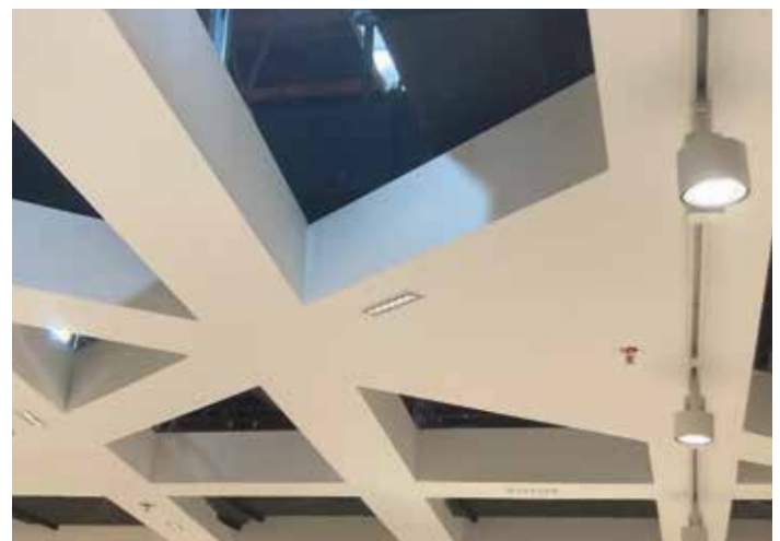
A close up of the architectural ribbons that form the striking new ceiling in VHM's front entrance.
